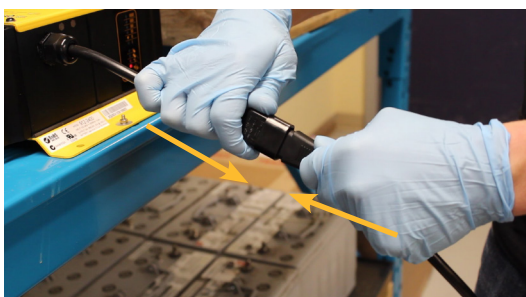
Figure 3: Reconnect AC power to the charger.
