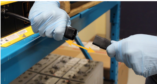
Figure 1: Disconnect AC power.
